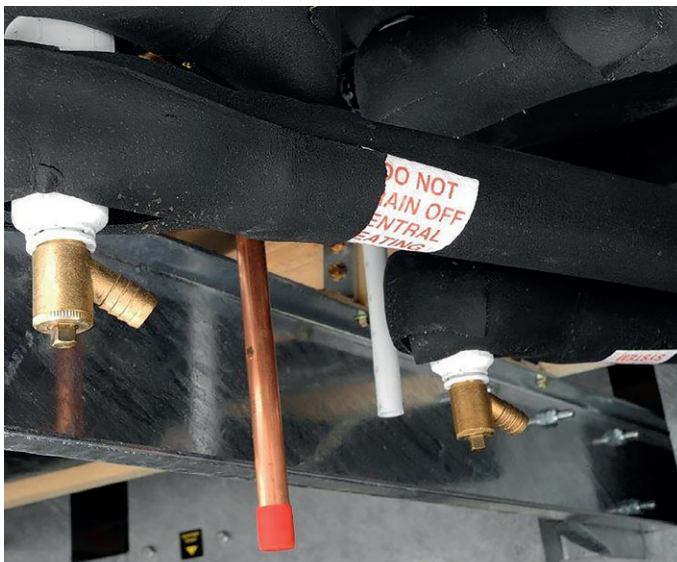
This photo illustrates the plumbing under the combi boiler of an ABI Holiday Home. The two drain cocks are for the sealed central heating system. Clearly marked with "Do not drain off central heating".
