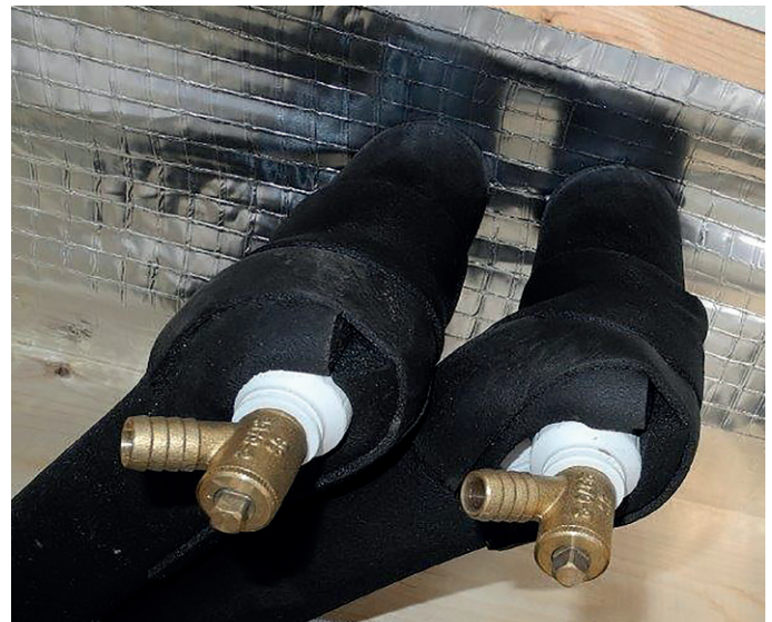
This photo illustrates the drain cocks for the fresh water system. This needs to be drained down for winterisation.
